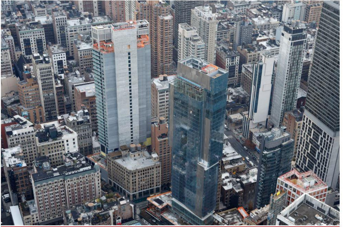
Ritz-Carlton Nomad during construction in 2020.
